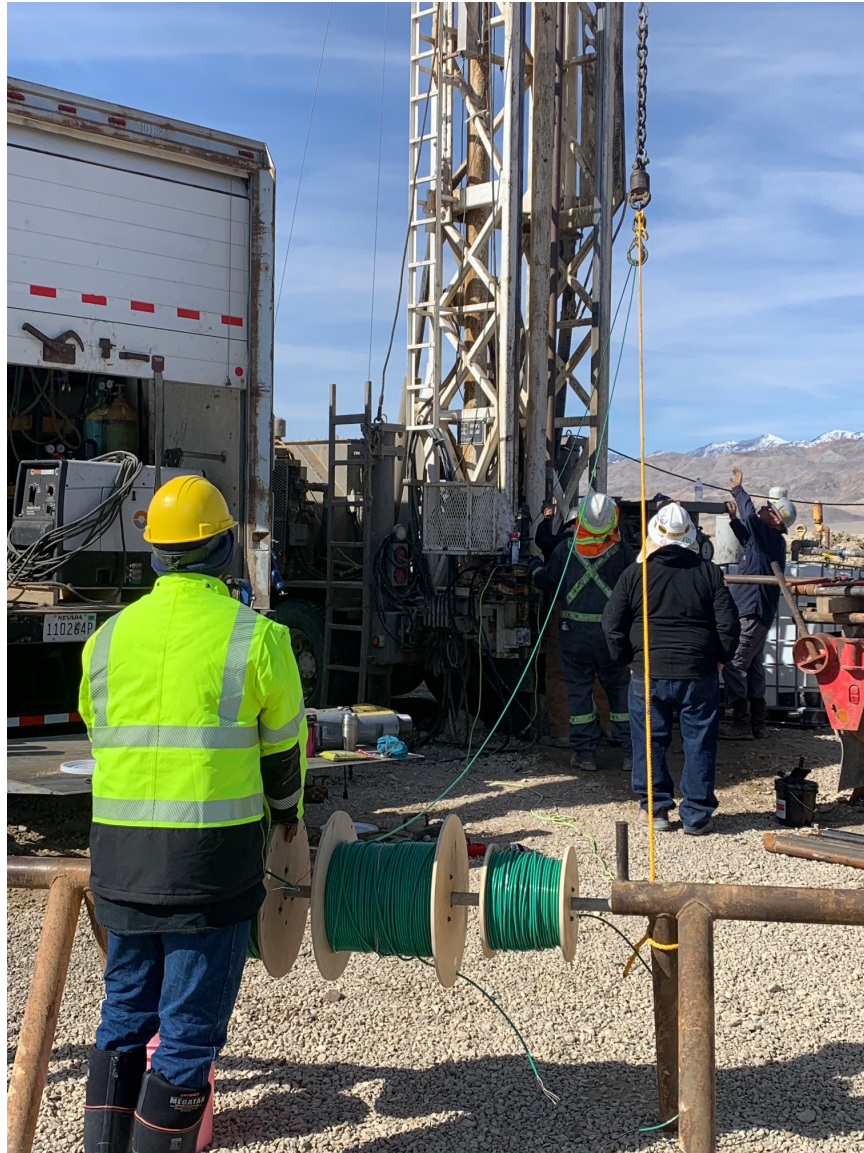
VWP Installation in DH-1A at Clayton Valley, Nevada (Fig. 1)
