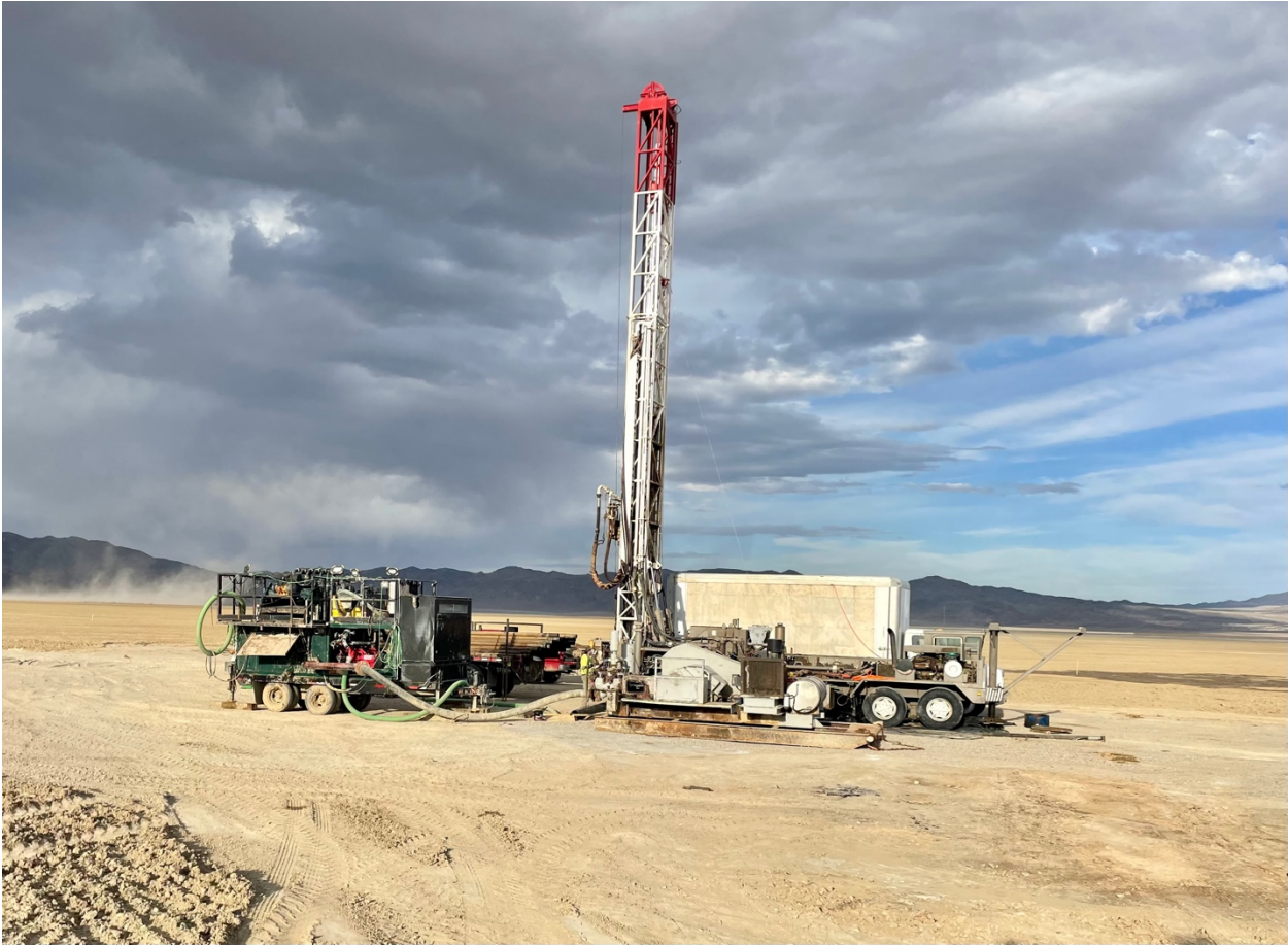
Figure 1: Clayton Valley Property Drill Set Up
